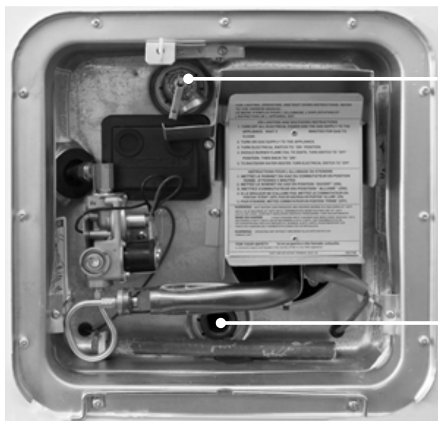
Pressure Temperature Relief Valve
